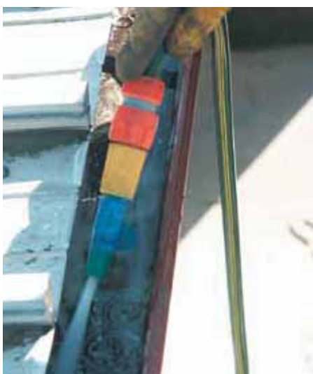
4) Rinse the gutter with water to soften and break up the dirt.
