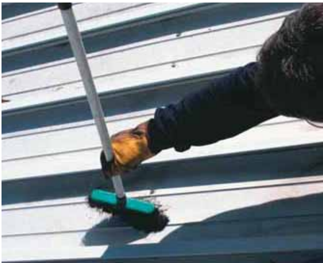
3) Use a soft bristle brush to sweep out the pans. Rinse with water.
