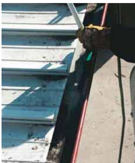
5) Use a soft bristle brush and sweep the dirt out. Rinse again.
