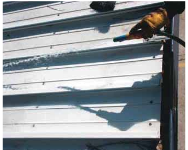
2) Use a hose to blow away twigs and soften hardened dirt.
