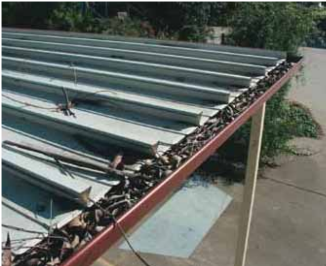
1) A typical suburban roof with leaf litter and dirt prior to cleaning.
